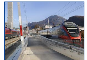
Railway Bridge Salzburg
