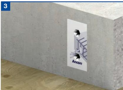
When the concrete has achieved sufficient strength, strike the shutter. Peel off or puncture the label to reveal the holes for the dowels. Where 'Q' versions are being used, the label should only be punctured enough to allow the dowel into the cylindrical sleeve to prevent debris entering the box section.
